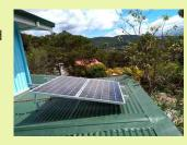
Sizing the solar array and the batteries required is complex. Detailed analysis of your requirements will be needed to provide for your minimal critical needs. You'll also need to rewire your main electrical panel to isolate the "critical loads" so that only those are provided power in an outage. This means that your well pump, refrigerator and a few lights are provided power while your air conditioners and TV and other non-essential loads are not.
